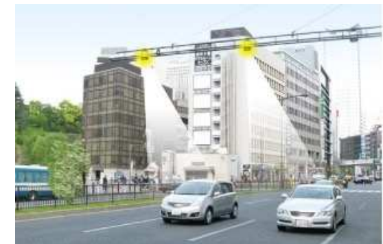
Infrared beacons (Ordinary trunk roads)
