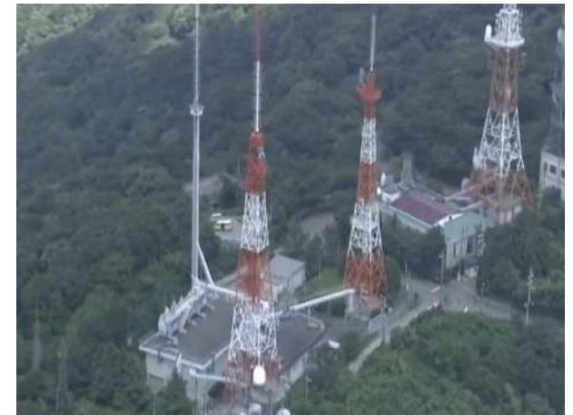
Broadcasting transmitting station
