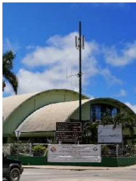
“Early Warning Siren system” using Radio EWBS
