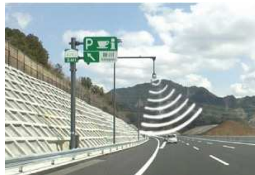
Radio wave beacons (Expressways)
